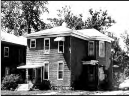
Before — original porch missing.
