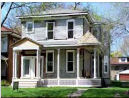
After — new porch based on original.
