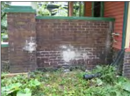
Improper repointing damages masonry and diminishes curb appeal.
