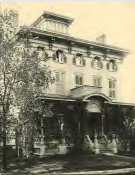
Historically, such items as shutters, porches and landscaping were used to enhance energy efficiency.
