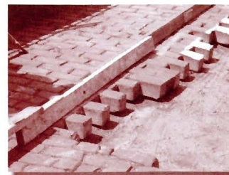
Example of "toothed" edge after removing bricks (photo by Jason Swisher)
