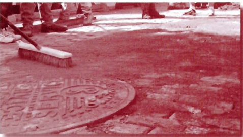
Preparing to brush in the grout (photo by Jason Swisher)
