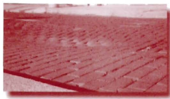
Collapsed area of brick street (photo by Jill Downs)
