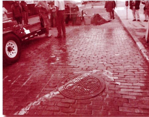
Completed repaired brick surface (photo by Jason Swisher)
