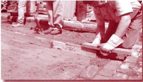
Screeding of the sand layer (photo by Jason Swisher)
